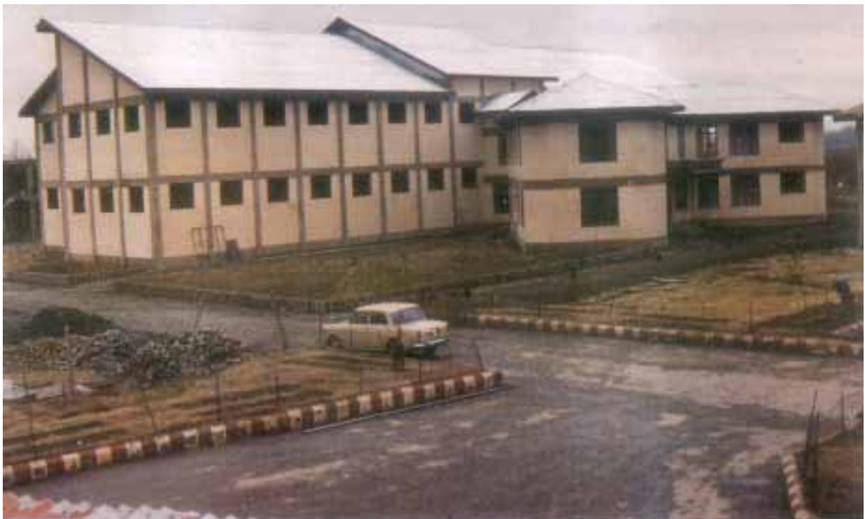
Central Record Room: Revenue Complex, Jammu and Kashmir
