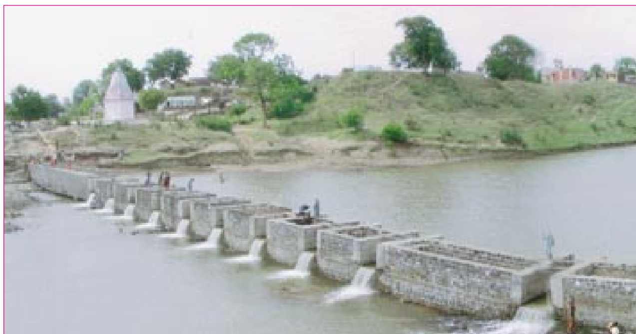
Harvesting of water through a stop dam
