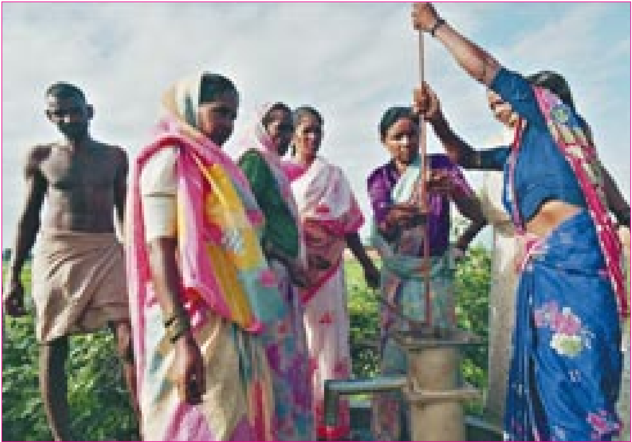
Women mechanics repairing a handpump in a community maintenance project
