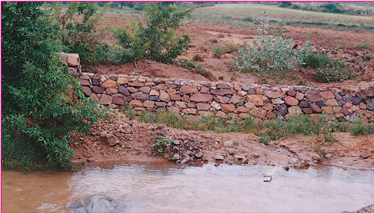
Rock Filled Dam
